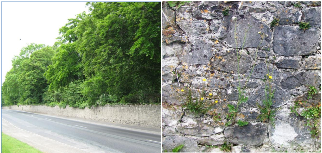
Fig. 7. Left, wall of Donaghcumper Demense. Vegetation obvious on top from Demense side but path side has probably been sprayed to keep it clear of vegetation (photo, Celbridge Walking Trails). Right, vegetation growing in cracks and gaps of masonry wall (photo, Caitriona Maher).
